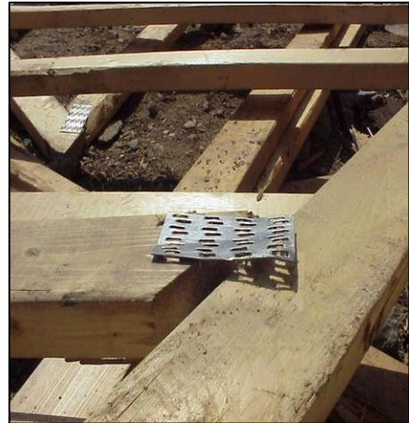
sink that conducts the heat of the fire to the wood destroying the bond between the gusset plate and the wood. *The gusset plates will penetrate the wood anywhere between 1/4 to a 1/2 inch.* In addition to acting as a heat sink, they are also known as the weakest point of the support system.
