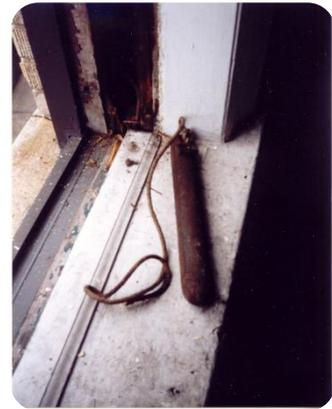
The cast iron weight averages around 2" in diameter, 10" in length, and can weigh as much as five pounds. The weights design and shape allows it to ride up and down in the vertical channel or pocket for the entire height of the window. In many older buildings, renovations have replaced the older wooden window sashes with newer and smaller replacement windows.
